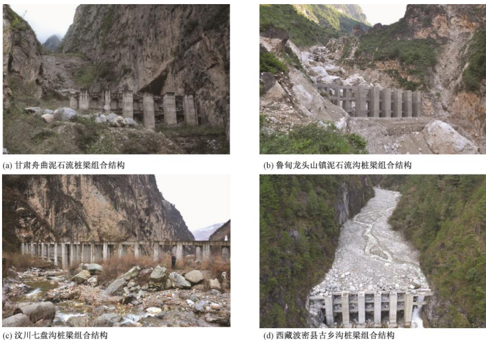
Figure 1. Photos of pile-beam composite structures
